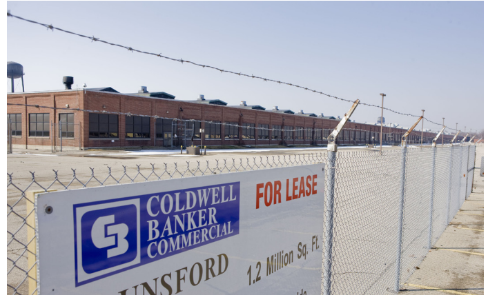
The BorgWarner Plant
